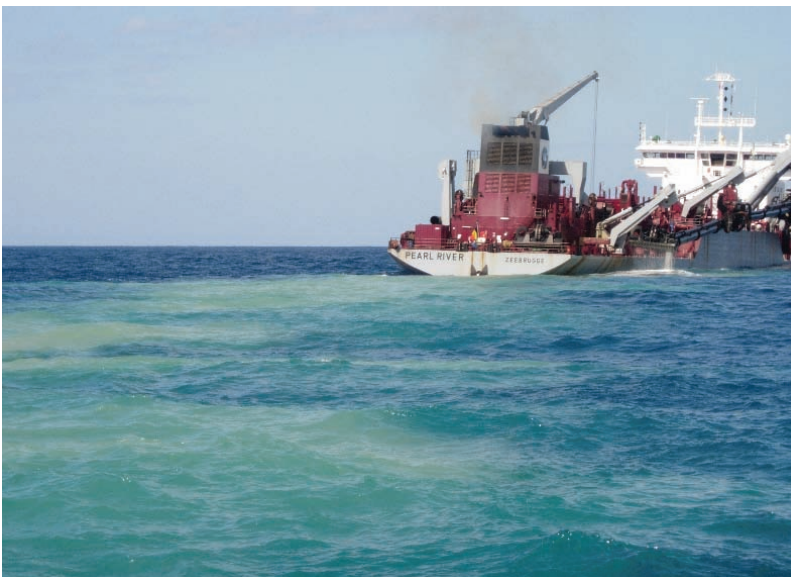
Figure 1.18 – Turbidity plume generated during sand transport from the dredging site to the nourishment site.
