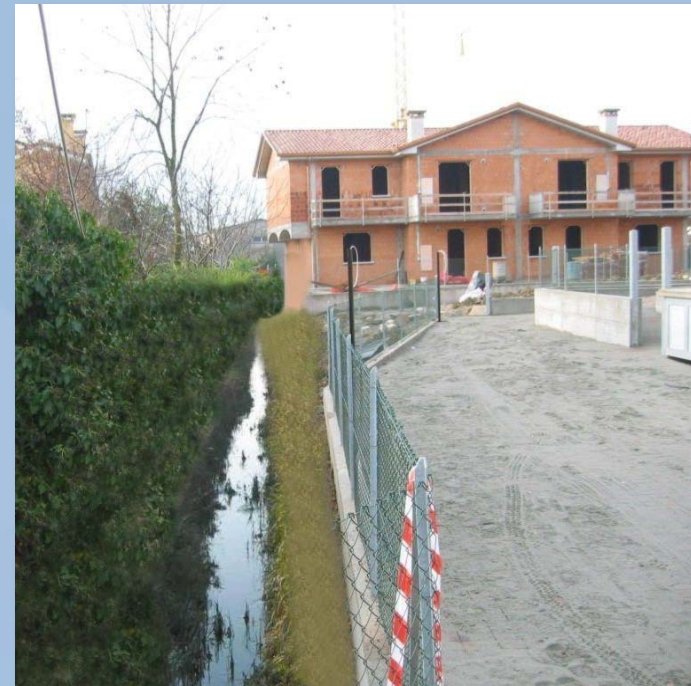
Ditch open = maintenance of drainage capacity
