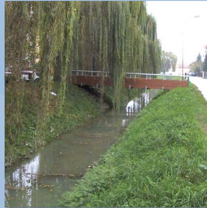
Net bridge = maintenance of hydraulic section
