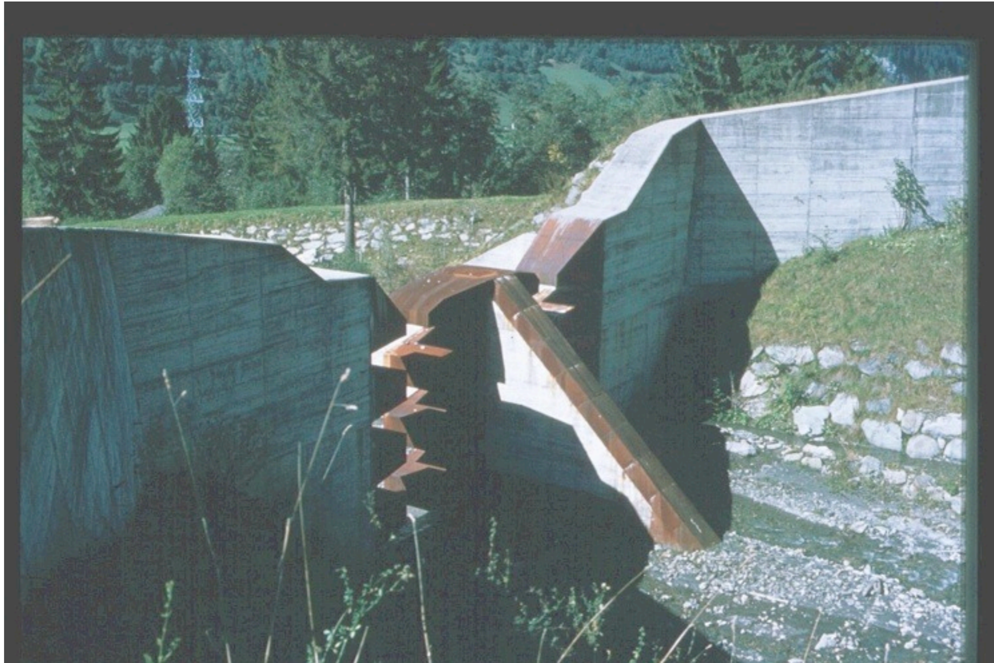
Courtesy del Prof. Aronne Armanini- Check dam with Debris Flow Breaker
