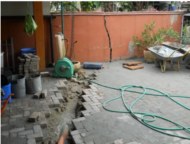
Fig. 4 – San Carlo (Sant’Agostino): ground ruptures and liquefactions affected farmed lands, paved roads and buildings.
