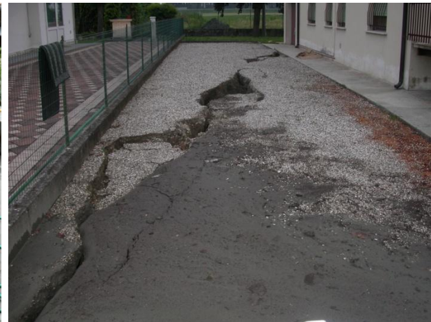
Fig. 4 – San Carlo (Sant’Agostino): ground ruptures and liquefactions affected farmed lands, paved roads and buildings.
