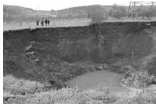
Figure 3 - Marcellina sinkhole (A. Colombi)
