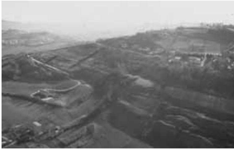
Figure 5.6 - Aerial view of the December 1982 Ancona landslide.
