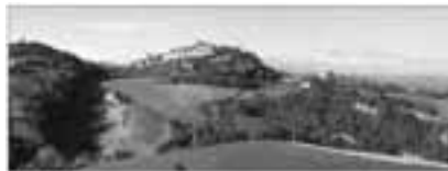
Figure 5.1 - Frontal view of the landslide area
