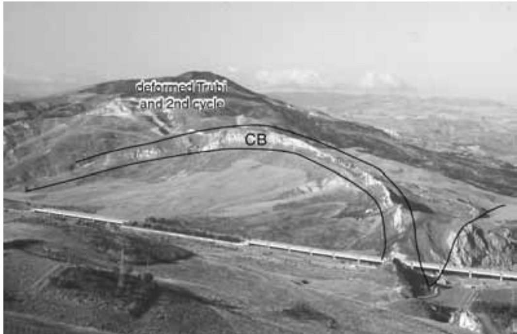
Figure 1.12 - Folded Messinian strata within the Corvillo Basin at the Cinque Archi motorway junction, looking east.
