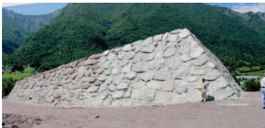
Figure 16 - Diversion cone placed near the top of the alluvial fan in the Rossiga Torrent, built to protect the hamlet of Galera.
