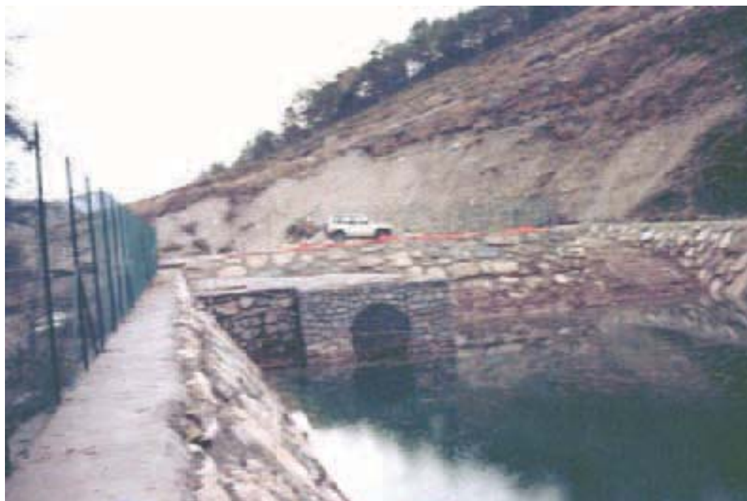
Figure 68 - The intake construction built after the event to allow a safe remedial work realization. The work is located at the left edge of the accumulation body, which has dammed the river bed. The water are collected from the Magnone stream and discharged downstream to avoid the erosion of the landslide foot.
