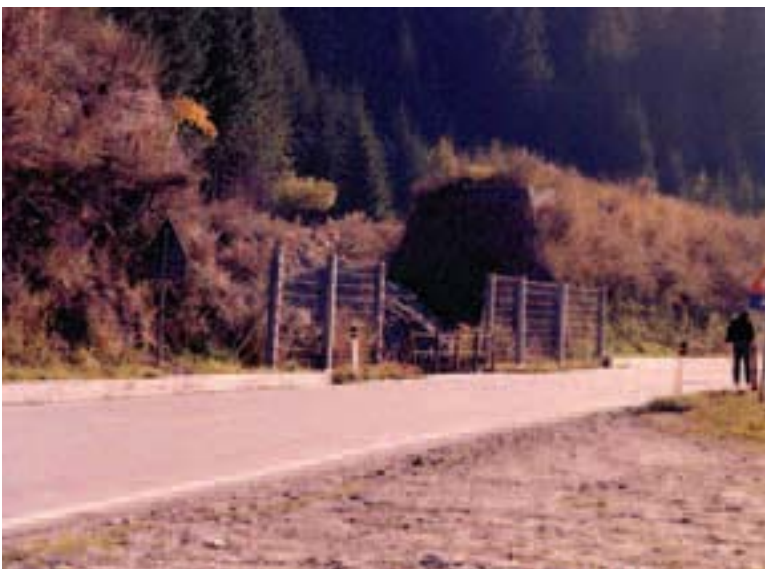
Figure 32 - The great reinforced earth wall which partially protects the road from the rocks falling from the lower parts of the Ruinon slope.
