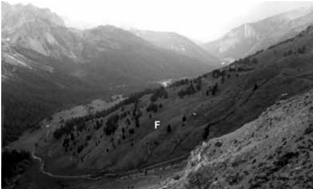
Figure 18B - Panoramic view of the S. Nicolò valley head from the mule track (altitude about 2200 m): a recent, fan sized, big slide, very likely due to deep seated detachment inside the present slope, can be observed
