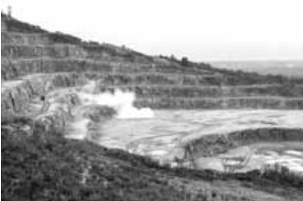
Figure 1 Stop 11 - General view of Botro ai Marmi quarry.
