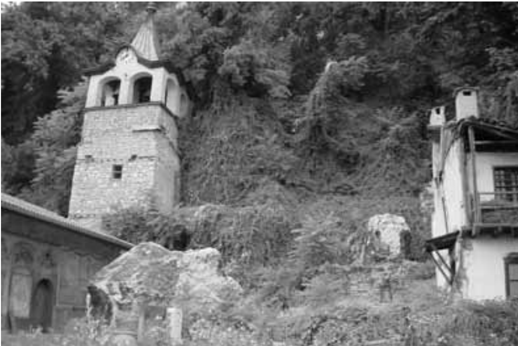
Figure 15 - View of the Monastery after the rock-fall
