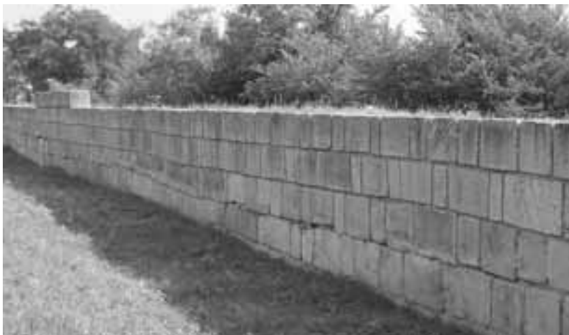
Figure 8 - Loess subsidence affected the Pliska walls
