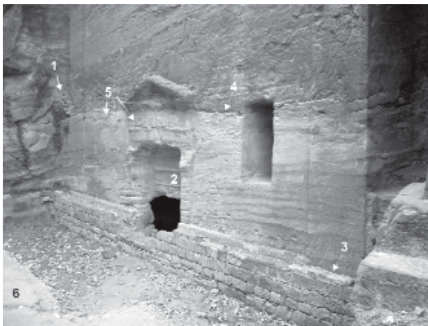
Fig. 15 – Recent excavation close to a Nabatean tomb, left downstream sector of the Siq, Petra. The highest alluvial patch (1) hints at a first alluvial event post-dating the monument; the monument weathering (2) likely pre-dates both a second alluvial burial and the Roman channel (3) construction; weathering also stresses (4) the top-surface of the second alluvial fill, preserved in some patches (5) hanging on the tomb facade. In the foreground (6) the modern valley floor.
