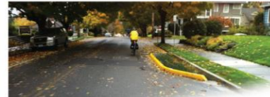
Curb Extension Bioswale Retrofit PORTLAND, OR
