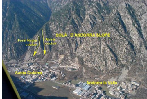
General view of the Sol`a d'Andorra with the rockfall active slopes and talus cones at their foot
