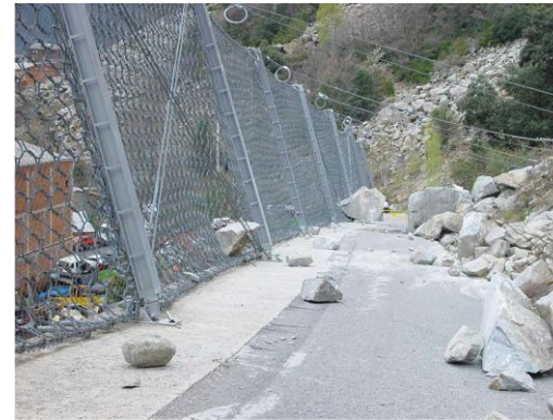
Two rock blocks of 0.25 and 4 m 3 respectively from the rockfall event of April 2, 2004, trapped by the protection fence of the Forat Negre basin
