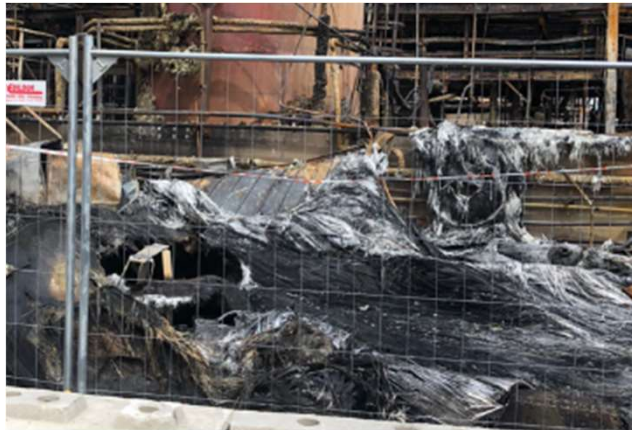
Collapsed Fiberglass tank
