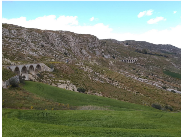
Fig. 15. Panoramic view of some of the viaducts that are still viable.
