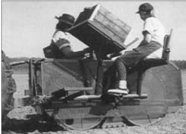
Figure 1: The Rotor cuttings transplanter used in the trial.
