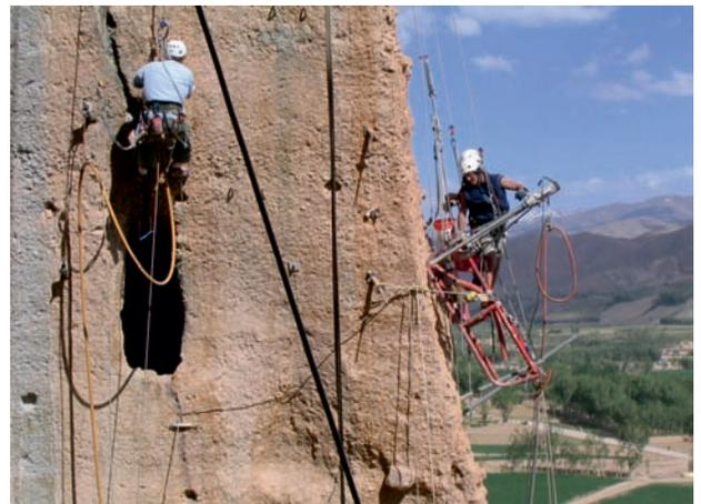
Fig. 10 – Consolidation works in the Bamiyan cliff.
