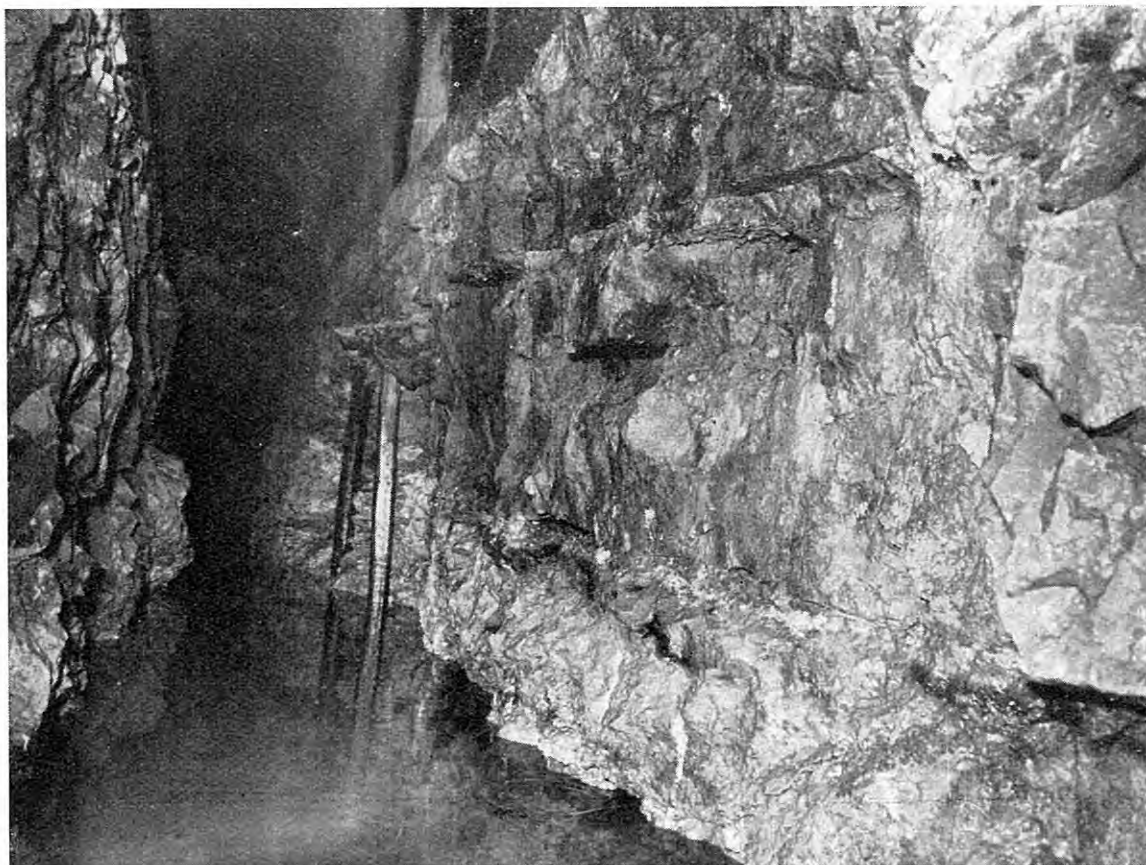
Fig. 11 - Draining shaft in limestone horizontal beds, where permeability derives chiefly from bed rock joints. The draining shaft was made at about 50 m below ground surface at the base of a well supplying water for industrial use in Mesagne area.
