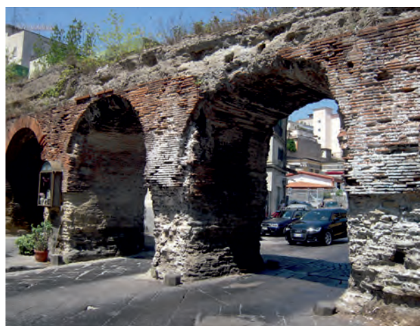
Fig. 10 — Ruederi dell'acquedotto Claudio (foto: P.M. Guarino). — Remnants of Claudio Aqueduct (photo: P.M. Guarino).
