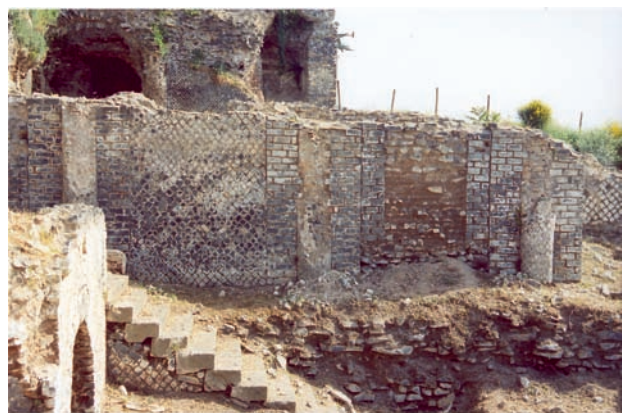
Fig. 10 – Barco Borghese, ambiente N. 191: parete divisoria con l'ambiente N. 159, decorata da semicolonne in muratura; da notare i passaggi originari tra i due ambienti tamponati in epoca successiva con murature in opera reticolata (foto M. Valenti). – Barco Borghese, room no. 191: dividing wall with room no. 159, decorated with masonry semi-columns; it should be noted that the passages between the two rooms were closed at a later date with an opus reticulatum wall (photo: M. Valenti).
